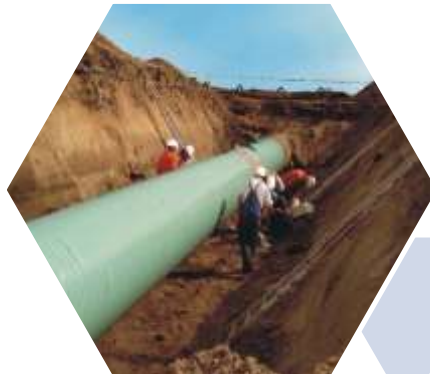
Pipe line Rehabilitation.
